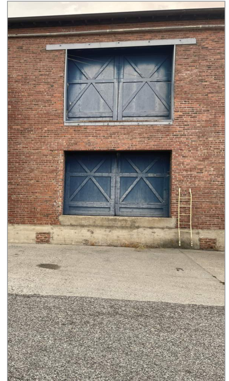
LOADING DOORS, BUILDING C
