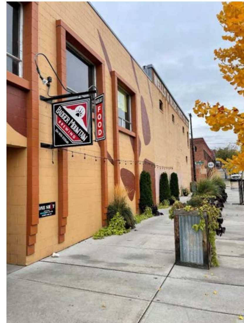
Figure 15: North Elevation of Buildings A and B
