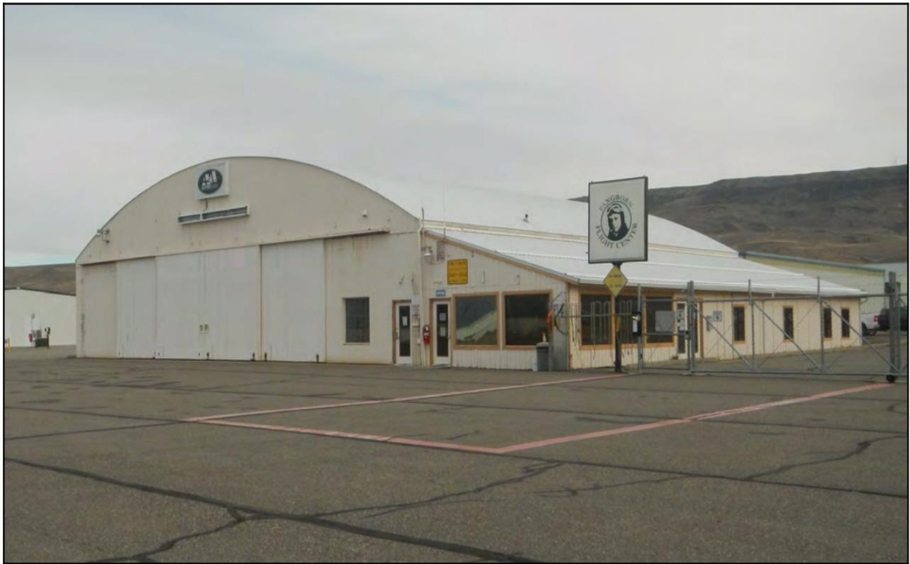
Figure 1: This photo is looking north at the front of the existing GA terminal building.
