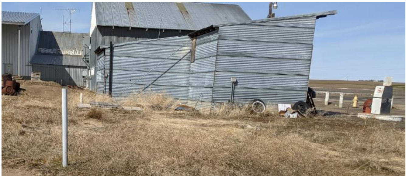
Photo 5 – View looking west towards east side of building. Reason for 2" gray pipe is unknown.
