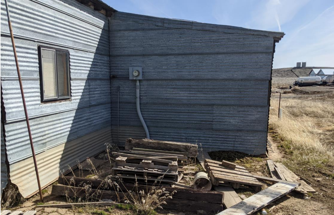
Photo 8 – View looking east at southwest corner of the building. Window appears to be for an office. Electrical service entrance still has meter installed.
