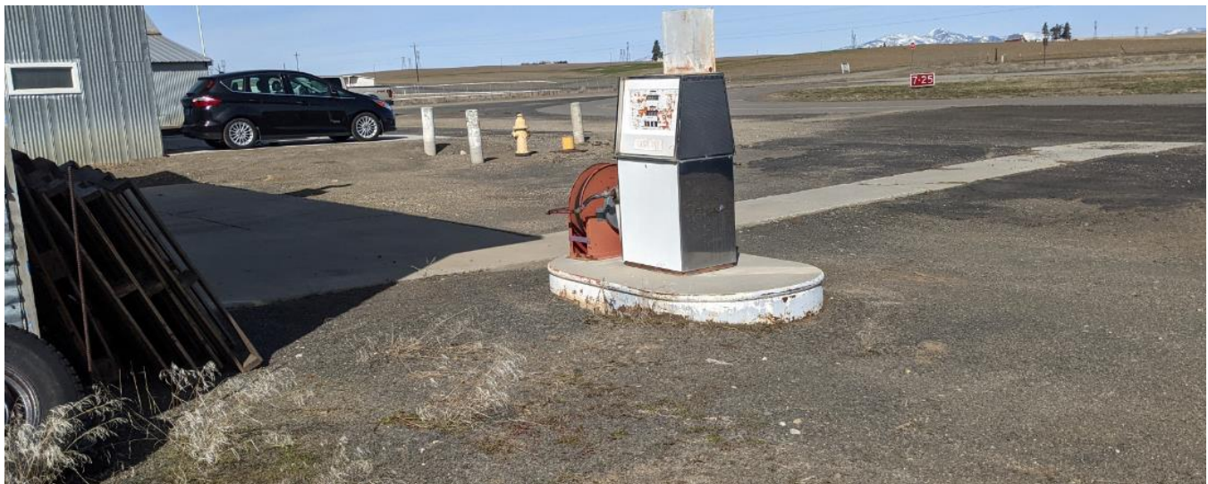
Photo 1 – View to the northeast showing fueling dispenser and concrete fueling ramp. Note the surfacing adjacent to the dispenser is gravel and the darker areas near the end of the concrete fueling ramp are either asphalt pavement or chip seal. There is a 20-foot wide concrete apron along the airside of the building. Note debris stacked against the building.
